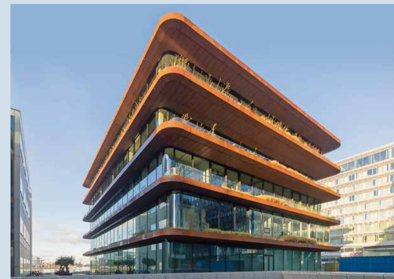
DANZIGERKADE 207 OFFICE AND COMMERCIAL BUILDING IN AMSTERDAM, Netherlands A complex glazing with curved corners and floating windows consisting of sun protection insulating glass GEWE-therm® sun.
