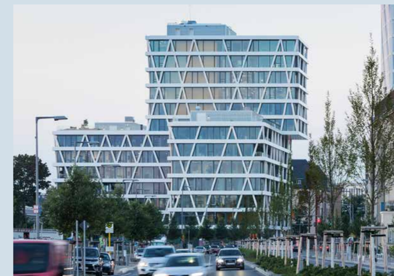
CORPORATE HEADQUARTERS 50HERTZ IN BERLIN A façade glazing variable in function and produced by SCHOLLGLAS by using GEWE-therm® consisting of GEWE®-safe and GEWE®-dur H and GEWE®-safe consisting of GEWE®-dur and GEWE®-dur ESG-H with screen printing.
